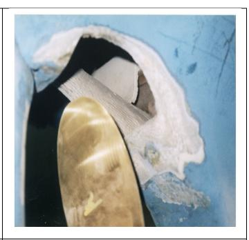
Lower portion of aperture ground out with the same amount of clearance
